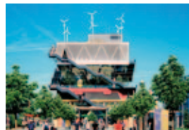
MVRDV_Expo_VR_72.jpg Expo 2000, Hannover Credit: © Van Reeken
